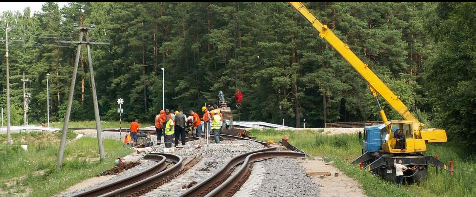
Oprava mostu / Bridge reconstruction / Remont mostu
